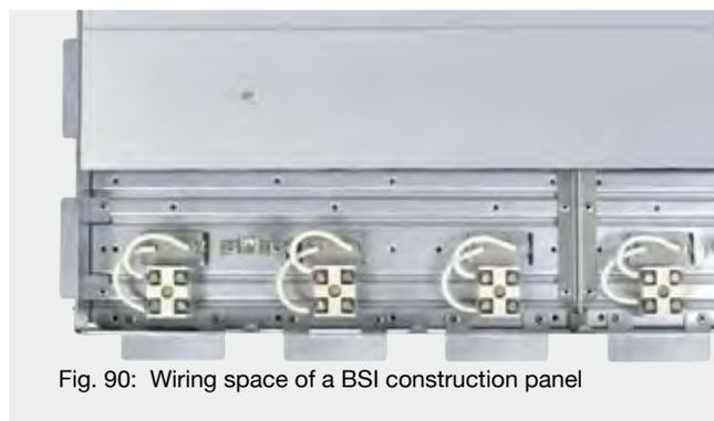
Fig. 90: Wiring space of a BSI construction panel
